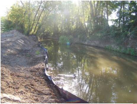
Canal at restoration segment
