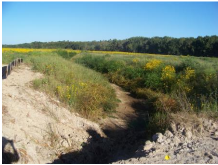
New meanders right after construction
