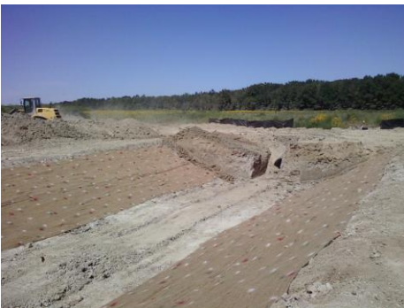
Erosion control blankets at the new meandering channel inlet
