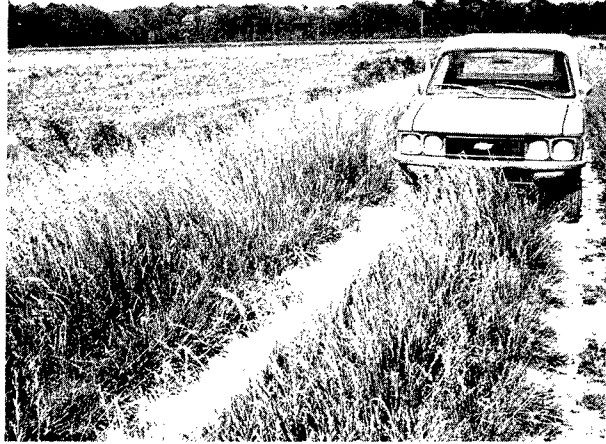
Fig. 2. Exterior levees constructed on Mingo National Wildlife Refuge have a top of at least 3 m with a slope of 3:1. These large levees readily support vehicles and heavy equipment and facilitate control of woody growth and muskrat damage.
